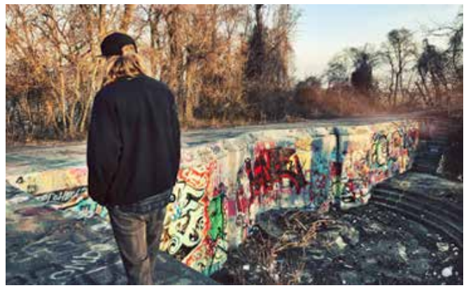
Battery McFarland (three 8-inch DC) with potential CDSG member.
