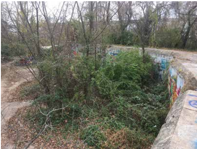
Battery Winchester (one 12-inch DC) emplacement.
