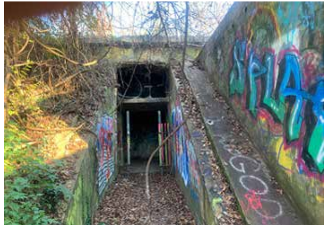
Battery McFarland magazine entrance.
