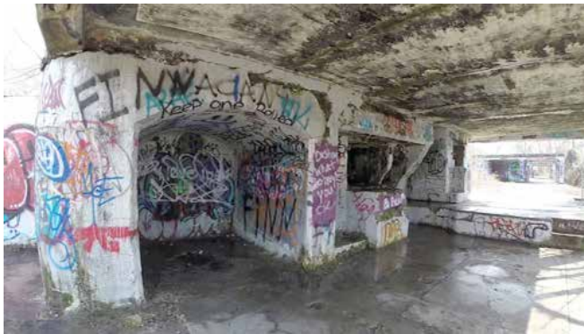
Battery McFarland shell lift and shot cart storage.
