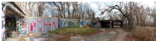
Battery McFarland emplacement No. 2.
